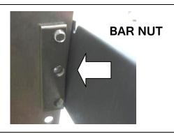
NUT BAR is installing when cabinet is not threaded to hold screws.
